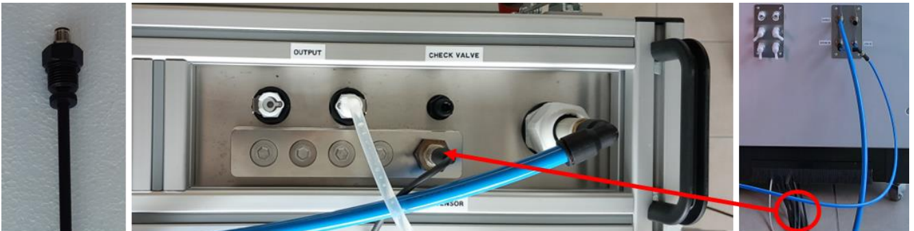
Fig. 19 Temperature sensor installation.
