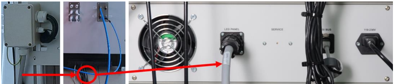
Fig. 14 LED panel installation.
